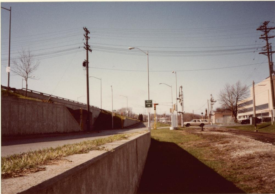
Highland Avenue exit from Campus Drive westbound
