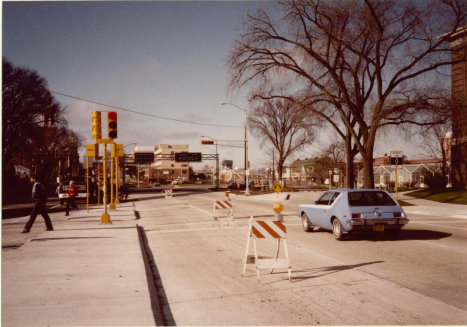
Campus Drive - University Avenue intersection East of the subject looking west
