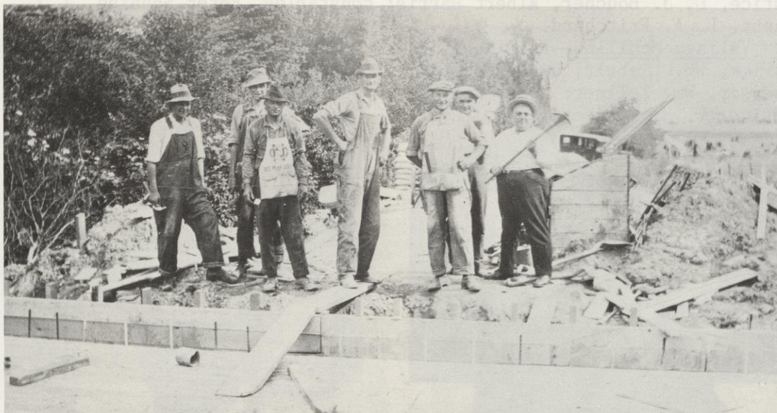
The "Bridge Gang" building Riverside Bridge
