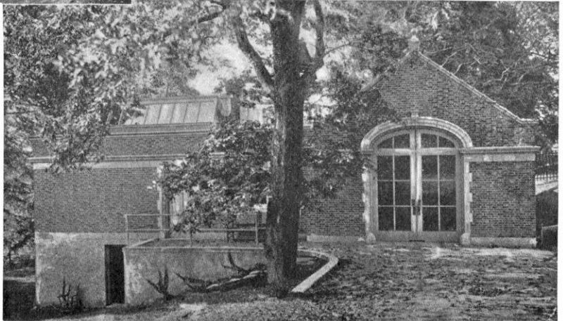
A GARAGE OF TAPES-TRY BRICK BUILT UPON A HILLSIDE WHICH INCORPORATES A SPACIOUS SQUASH COURT AND GOOD-SIZED GUN ROOM.
