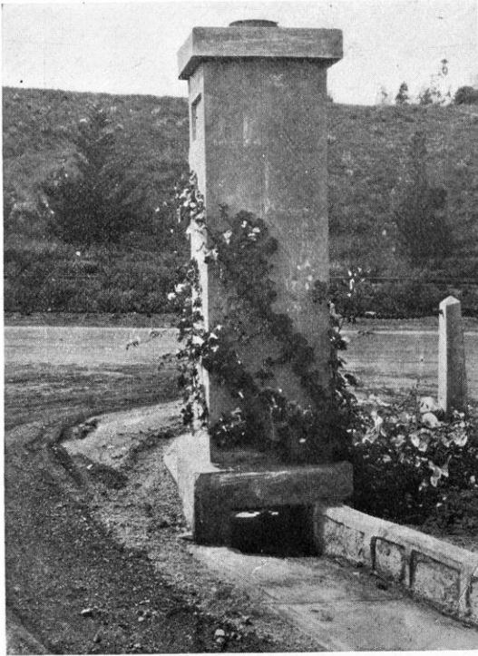
CONCRETE PILLAR AT THE END OF CURBING SERVING AS A BRIDGE.
