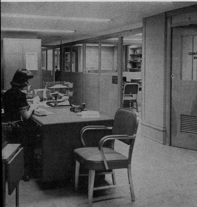
Old 14-foot-high rooms were sliced in half to form administrative offices below, and a series of study cubicles above.
