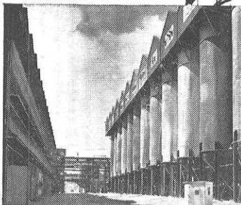
Settling tanks, where impurities are separated from sodium aluminate
