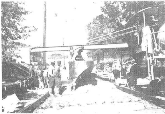
Applying fly-ash concrete.
