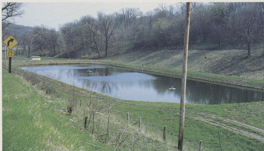
Sewage treatment lagoons like this one near Barneveld in Iowa County need to be sealed to protect the underlying groundwater.
