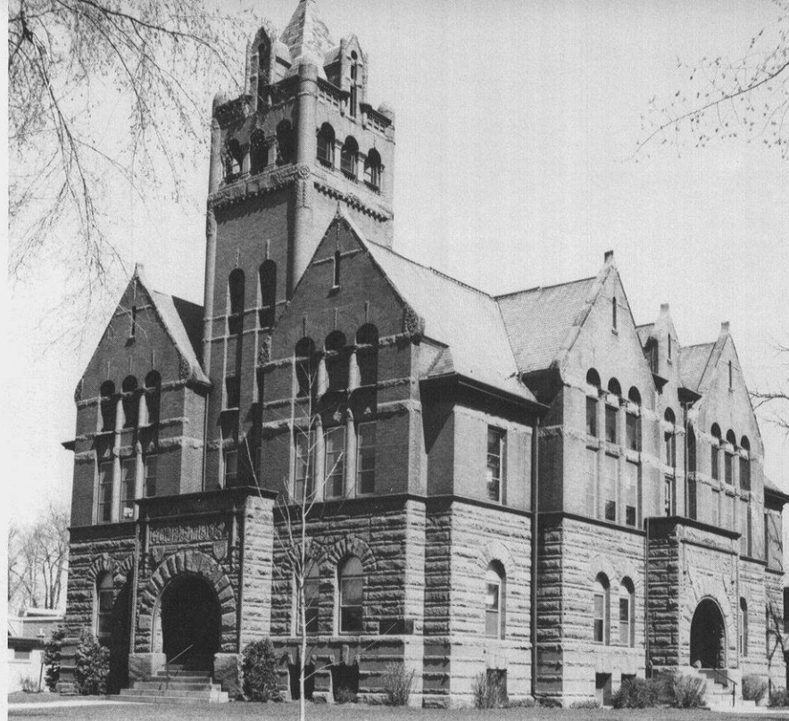
St. Croix County courthouse, 1899–1900, N. Hudson.
