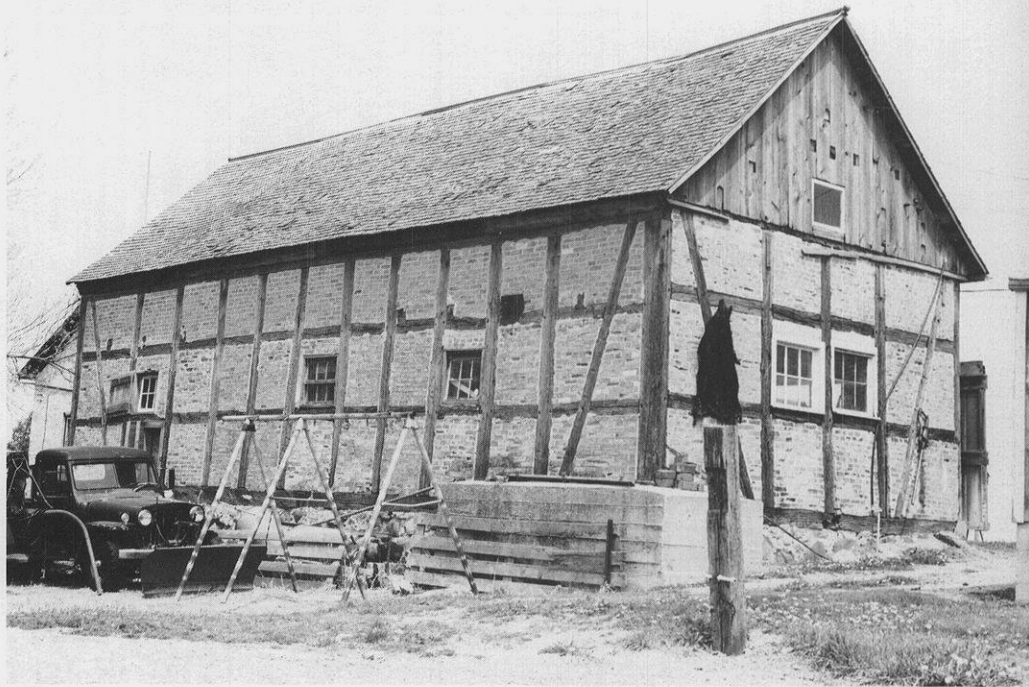
Immigrants from East Germany built hundreds of fachwerk structures in Wisconsin. The Kuenzi barn, shown here, from rural Dodge County, once had a thatched roof and has been carefully documented by the Historic American Buildings Survey program.
