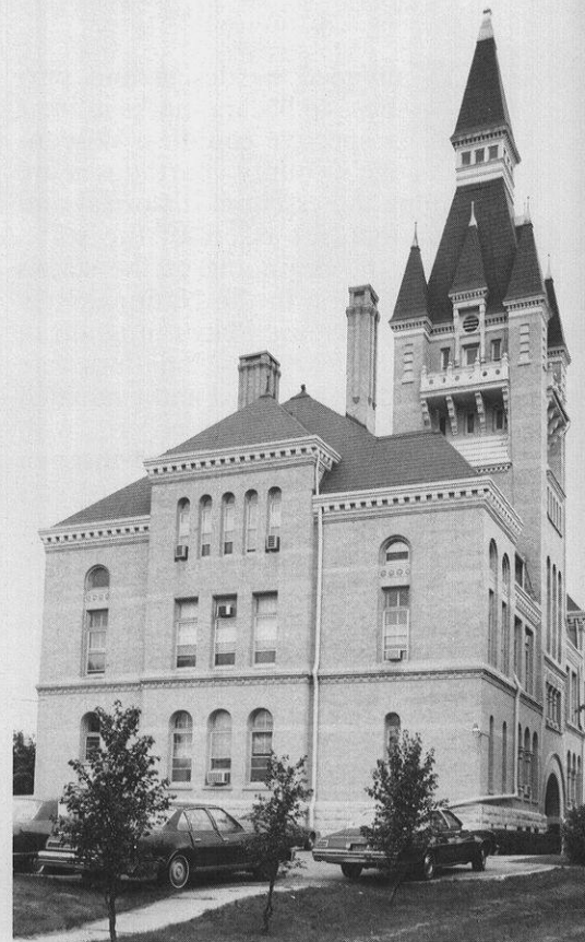
Washington County courthouse, 1889, West Bend.
