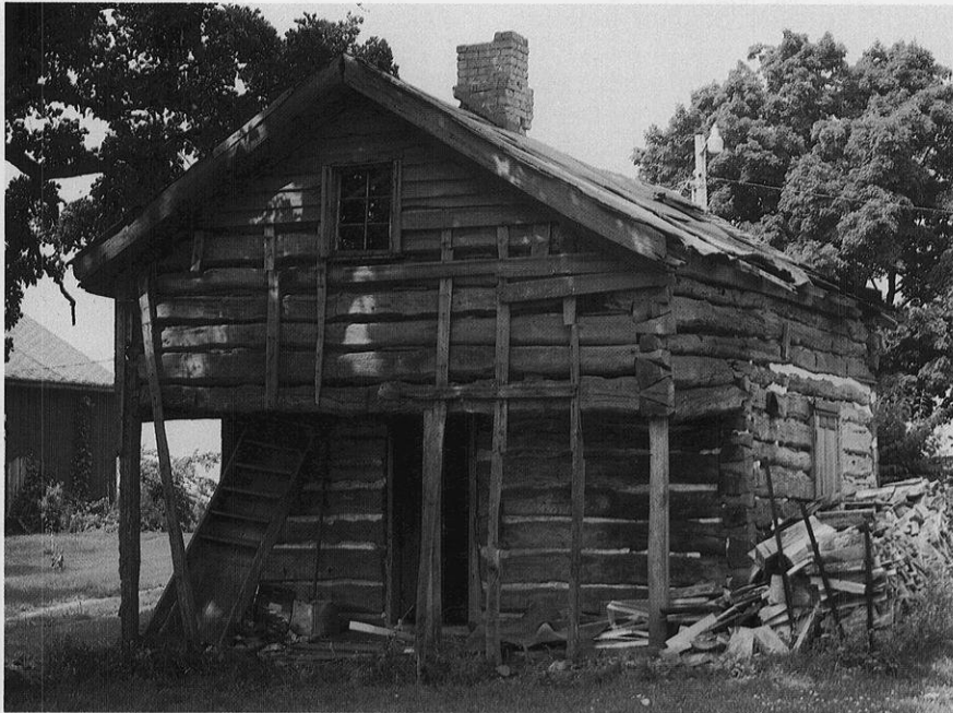
This rare example of a Norwegian loft house, with its exterior stairway to the projecting upper level, survives on a farm near Stoughton. It is a good example of an old world folk house form transferred to the early Wisconsin frontier.
