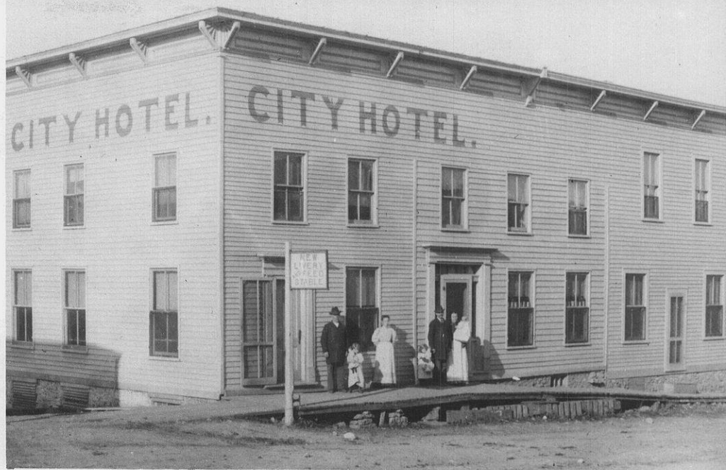
City Hotel, Shullsburg, Lafayette County. This historic photo was used to assess the integrity of the building today. The mining era intensive survey, conducted by the Southwest Wisconsin Regional Planning Commission, included the hotel in its survey.
