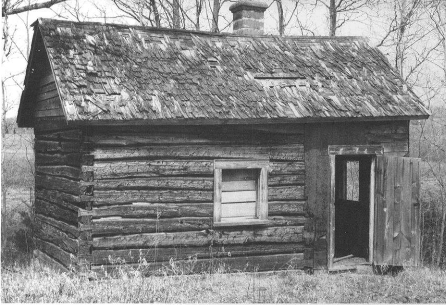
The Finns who settled in the northern reaches of Wisconsin's cutover country were highly skilled log builders. Finnish farmsteads typically included a sauna such as this well-crafted log structure with attached frame dressing room from Oulu Township in Bayfield County.
