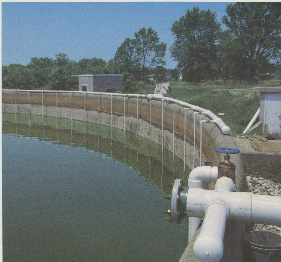
The special air supply for the three tanks now in use is pumped through a series of small pipes. Photo by John Beth
