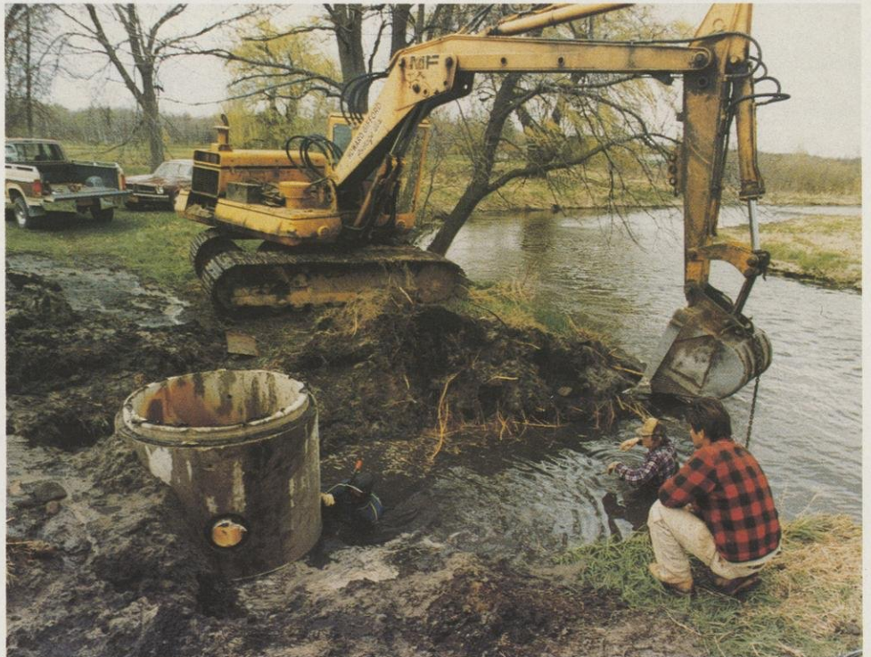
Installing the water pump intake structure on the Fox River. Photo by Don Schnering
