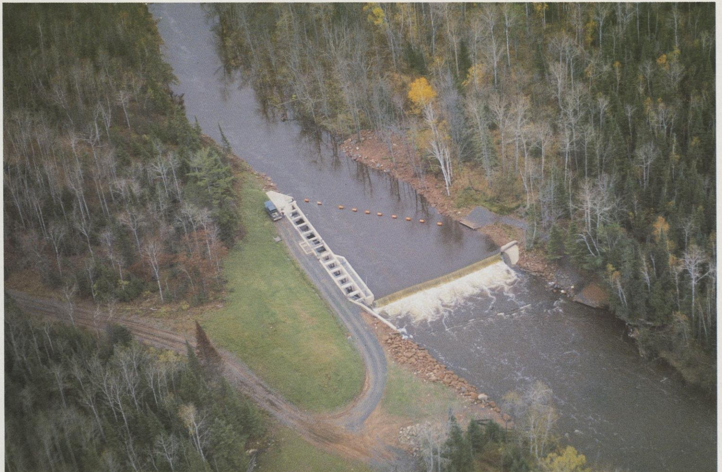
Wisconsin's unique fish ladder/ lamprey barrier on the Brule River. Photo by Fred Kruger
