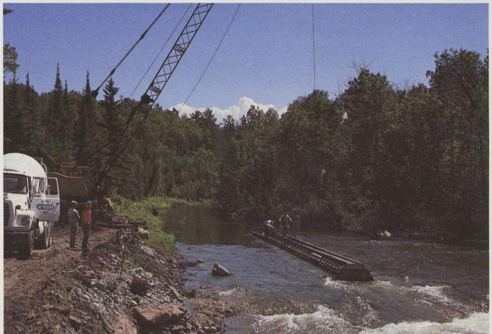
The first stage in building the fish ladder was construction of a cofferdam, which also served as the retaining wall for a temporary fishway. Photo by Dennis Pratt
