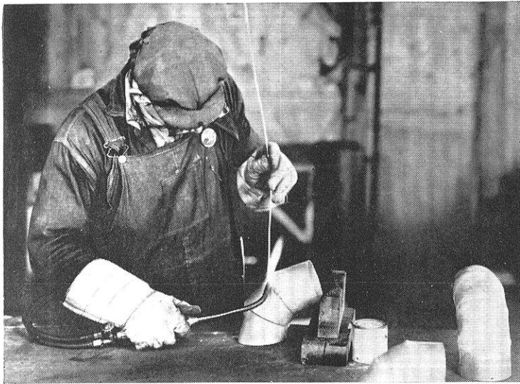
FEATHERWEIGHT PIPING —made by welding aluminum tubing. These fittings are to be used in a chemical plant.
