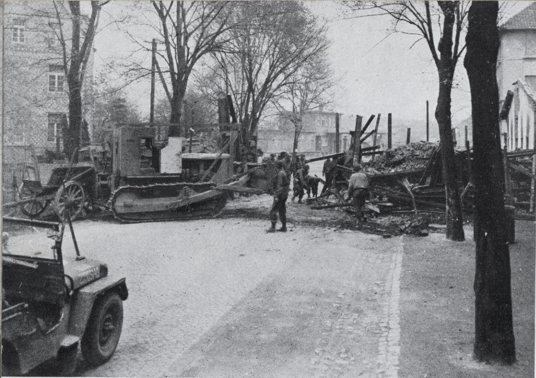
BARRICADES IN BRUNSWICK go down before blows of an engineer bulldozer.
