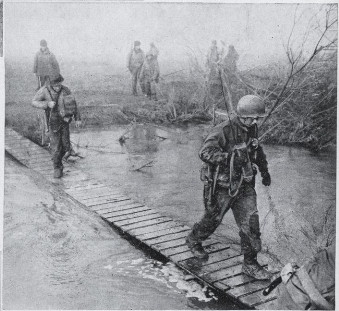
NARROW, PRECARIOUS footbridges served the assault waves.
