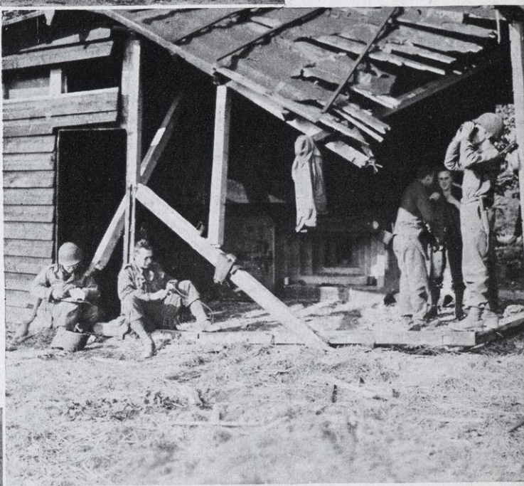
A "WOODEN" PILLBOX near Ottenfield, Germany. A shack camouflaged the concrete structure.
