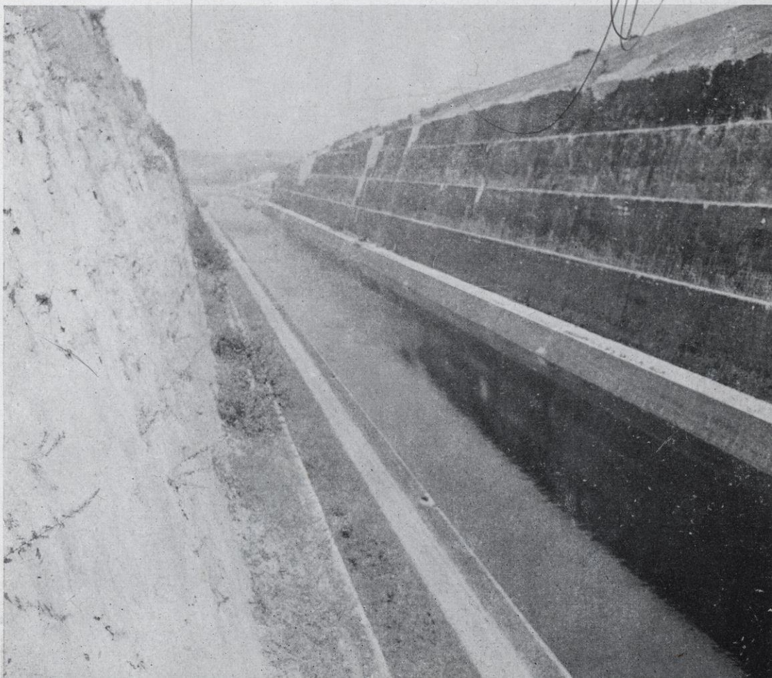
THE ALBERT CANAL near Fort Eben Emael, Belgium.
