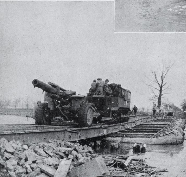
BIG GUNS NEED BIG BRIDGES. By H plus 24 engineers had a treadway over the river and the 155mm. howitzers were rolling across.
