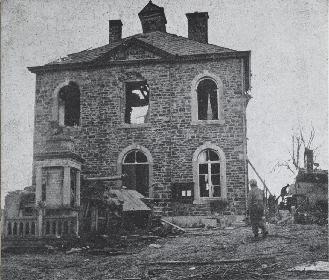
LA GLEIZE CITY HALL, just after the battle. Note destroyed German tank in front of the building.
