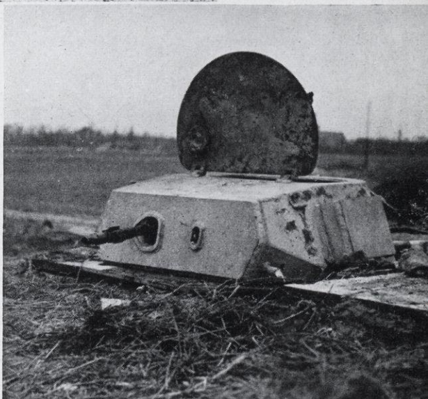
STRONG EMPLACEMENTS marked the German Roer line. This steel turret covered a roomy dugout.
