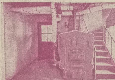
The boiler cellar. The stairs from the garage are at the right. The coal bin is at the left. The work room is seen through the door. The stairs from the greenhouse come down into it.
