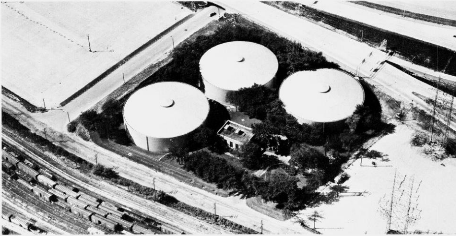
MENOMONEE VALLEY BOOSTER PUMPING STATION. EACH STEEL TANK HOLDS 6 MILLION GALLONS OF FILTERED WATER.
