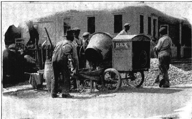
Rex Mixer on a Modern Construction Job
