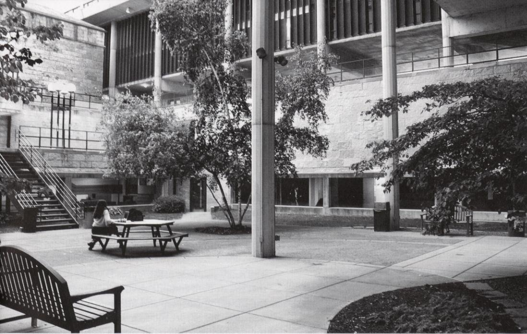
The center of the building is features a courtyard, which some consider to be a bit of an “intimidating” place to study.
