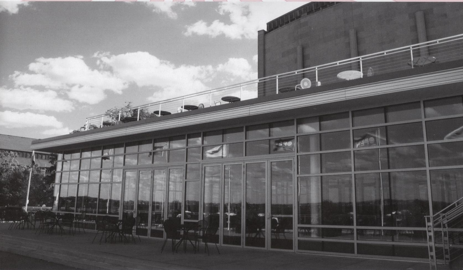
The Sunset Lounge in the renovated Memorial Union.
