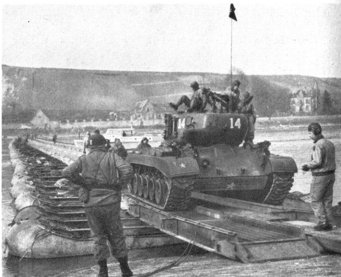
45-ton M-26 tank being guided across the specially designed 912-foot treadway span constructed by the 1st Engineer Battalion at Oppenheim
