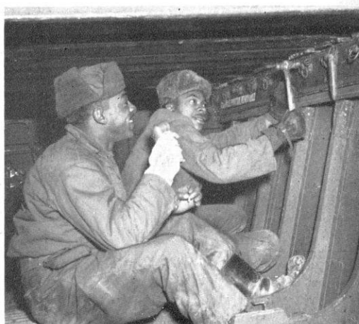
Two members of Constabulary engineers pounding iron pegs into place to secure bridge for troops
