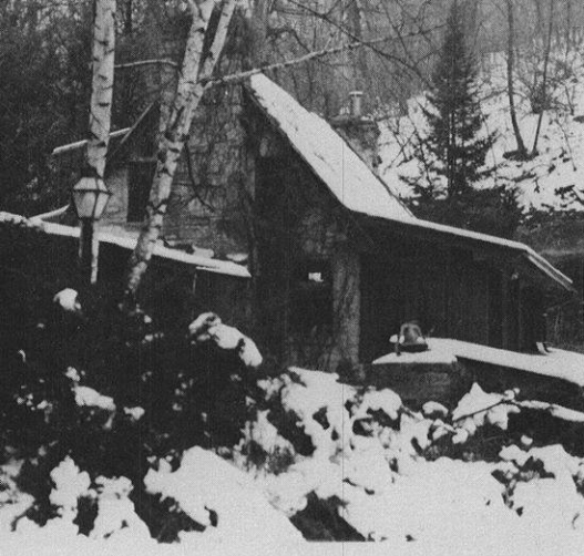
The Johansens' Blue Mounds home was constructed of wood and locally quarried limestone.
