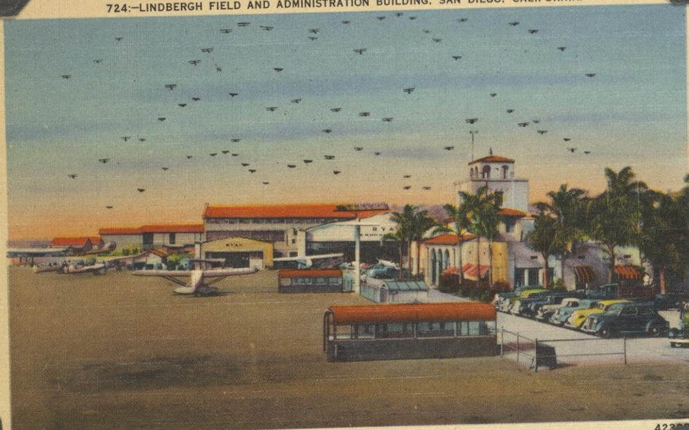
724:-LINDBERGH FIELD AND ADMINISTRATION BUILDING, SAN DIEGO, CALIFORNIA.
