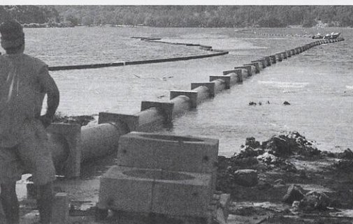
Contractors spent a week and a half attaching blocks as 4,150 feet of pipe was extended into the lake.
