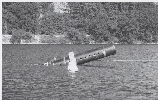
Holes in the 50-foot intake were aligned horizontally before it was sunk to the lake's deepest spot. The pipe now draws water just above the lake sediment.
