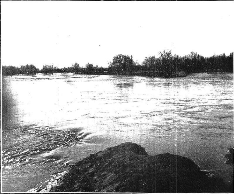
Fig. 4—View along Axis of the United States Government Levee Just South of Portage, Showing the Crevasse Made by the Wisconsin River Flood of April, 1900.
