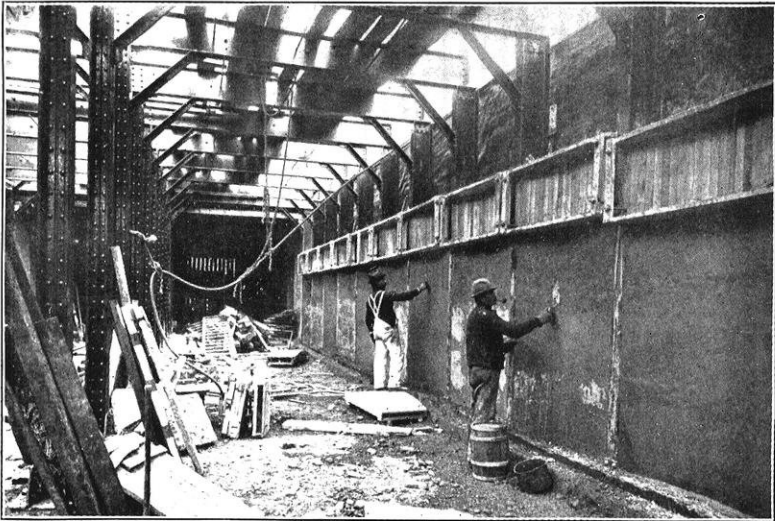
Fig. 3—Finishing Concrete Side Arches.
