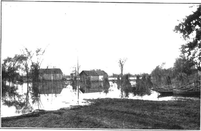
Fig. 3—Highway and Farmhouses Submerged by the Breaking of the Caledonia Levee in the City Limits of Portage.
