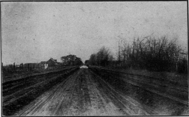
Trench thrown out with a road machine and sand ready to receive broken stone. This system of laying stone or gravel in a trench should be followed on all roads whether a steam roller is used or not.
