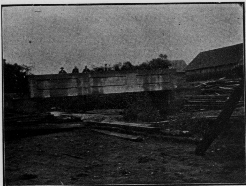
Reinforced concrete girder bridge, 36 feet clear space, town of Sand Creek, Dunn county. Contract price, $1,147, for bridge and abutments complete. Built under plans and specifications of the Highway Division.
