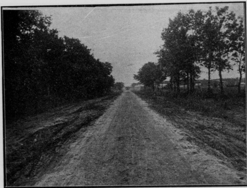
Stone road nine feet wide, Almond, Wis. Built under the plans and supervision of the Highway Division.
