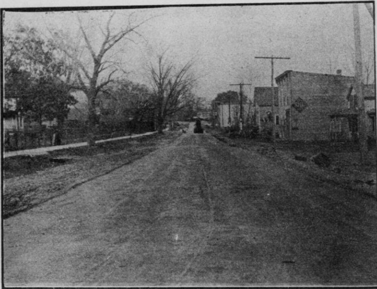
Street to depot, Hartland village, Waukesha county. Built with crushed gravel from local pits. Plans, supervision and machinery furnished by the Highway Division.
