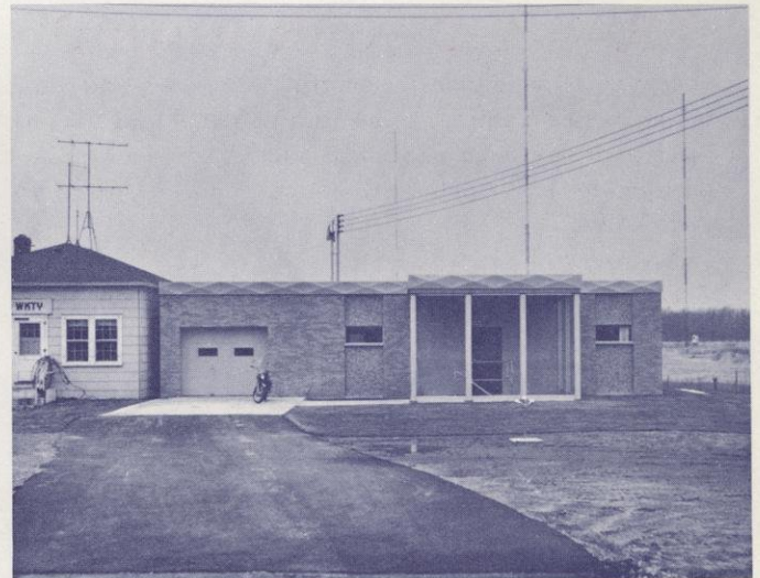
WKTY NOW PROTECTED STATION
