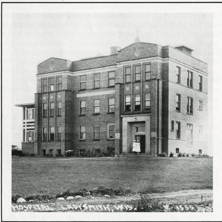
In the early 20s the east wing of St. Mary's Hospital was enclosed to provide a chapel and a pediatric facility.
