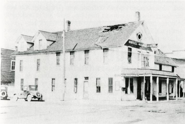
A fire in July of 1927 burned a hole through the roof of the Manley Hotel. A second fire, 10 weeks later, caused additional damage. The building was razed and a filling station was built on the lot.
