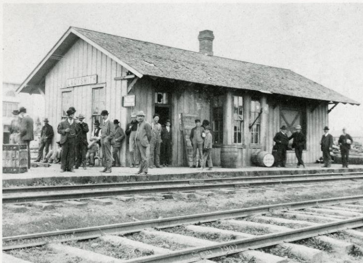
The first depot at Flambeau Falls was built in 1885 or 1886 by the Minneapolis, Sault Ste. Marie & Atlantic Railway. Smaller than the depot at Bruce, it was similar to the depot at Glen Flora. It was showing its age when this photo was taken in 1901.
