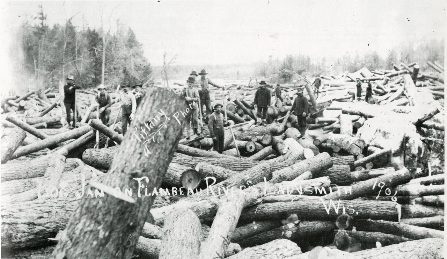
This Tiffany Studio photo is thought to show the log jam on the Flambeau River at Little Falls in late April of 1906. An estimated 1.5 million feet of logs were hung up in the center jam at the rock in the middle of the falls. The logs belonged to the Menasha Wooden Ware Co. With assistance from the Daniel Shaw Lumber Co. crew, the jam was broken on April 30 using large quantities of dynamite. There also was a log jam at the MWW Co. piers in Ladysmith that spring.
