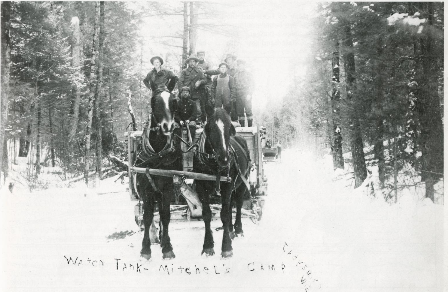
The water tank and crew from Mitchell's Camp near Ladysmith is pictured in this photo by Tiffany Studio. The ruts made by the runners of the logging sleighs were iced with water from the tank. The sleigh in the background probably belonged to the photographer.
