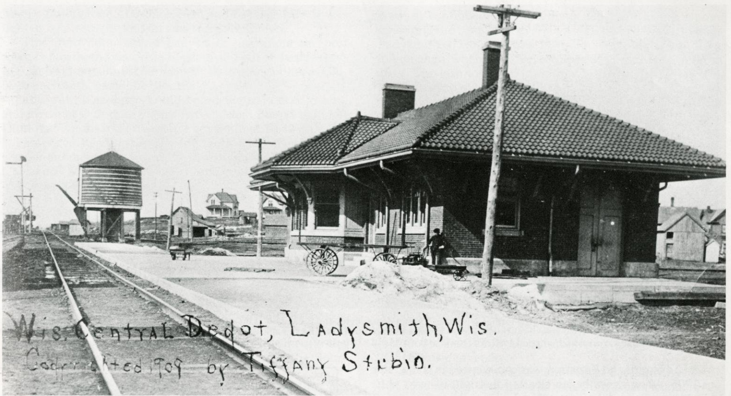
The Wisconsin Central depot was built at Ladysmith in 1906. The depot platform blocked Miner Avenue. The handsome brick structure was moved with horses in 1911 to its present location at the crossing of the two rail lines. Note the water tower and semaphore signal in the distance.
