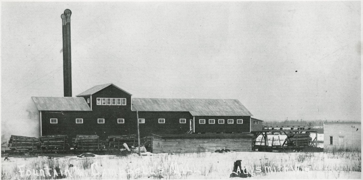
This view looking north shows the Fountain-Campbell Lumber Co. mill in Ladysmith, located near the present home of Mrs. Robert Goffin. The hot pond is at left, adjacent to the sawing room. The lath mill is at right. The twin stacks are for two boilers housed in a separate building to the north.
