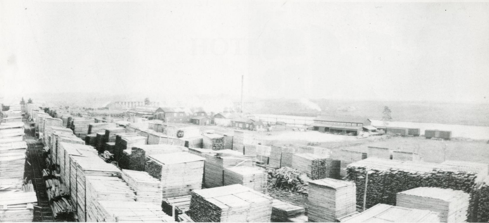
smokestack. The planing mill is at right. Lumber was piled from the mill north to Corbett Lake. Lumber wagons, pulled by horses rode on miniature rails.
