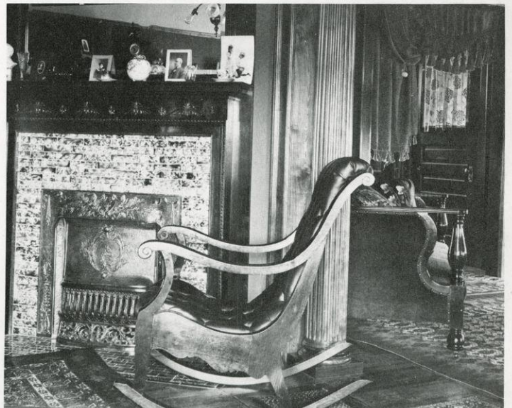
The fireplace in the R.S. Johnson home was designed with ceramic tile and copper. The oak mantel and carved pillars are examples of the woodwork throughout the house.
