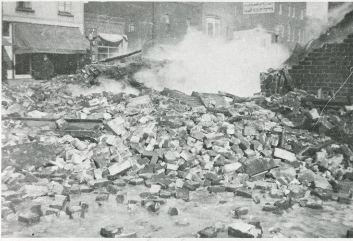
The smoldering ruins of J.W. Fritz's Pioneer Store in 1934. The building was occupied by Louis Cohen at the time of the fire.
