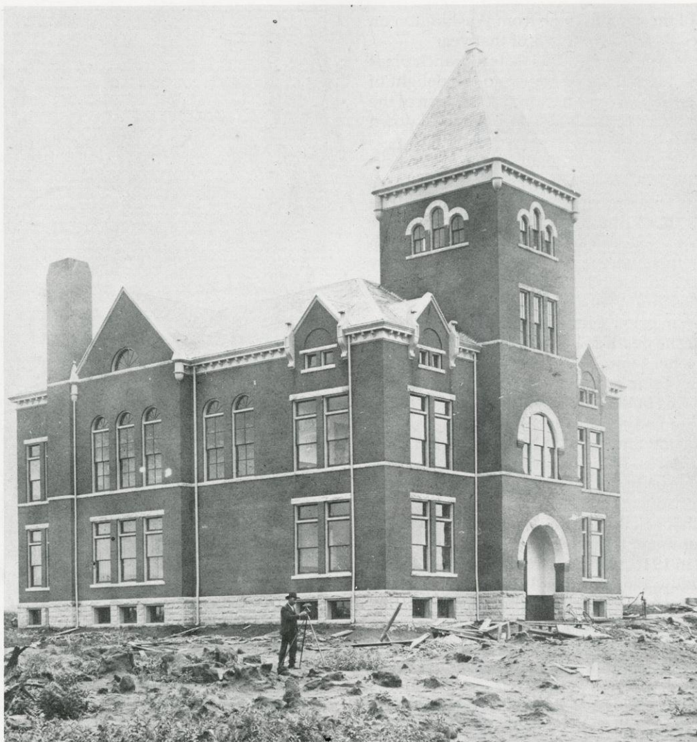
The Gates (Rusk) County Courthouse was nearing completion in the spring of 1902 when this photo was taken. The courthouse cost $25,000 plus $2,000 for the furnishings.
