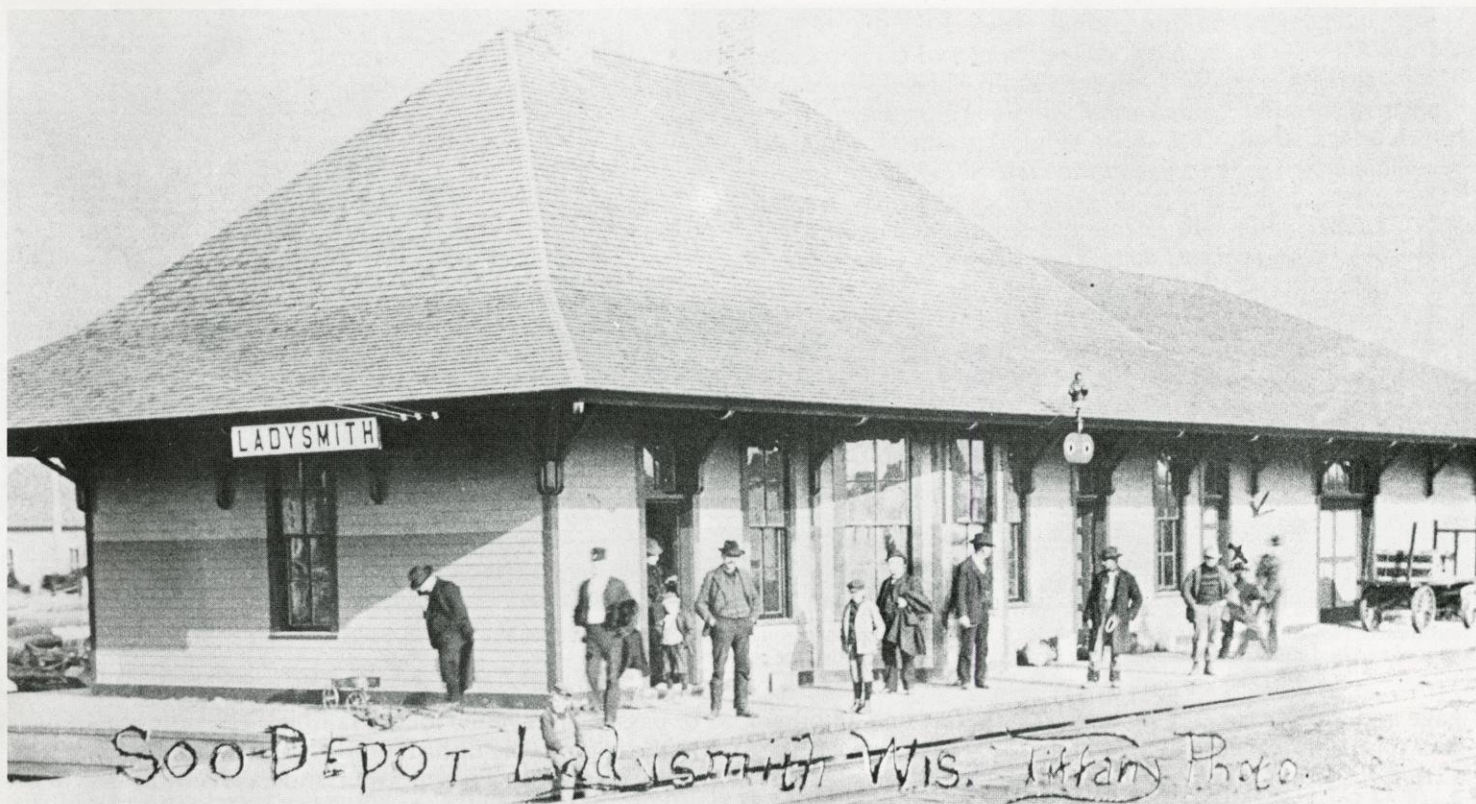
In 1904 the Soo Line built a new depot east of the first depot. It resembled the depot at Bruce. The high roof was later modified. The depot was moved in 1911 to its present location, where it serves as a freight house.
