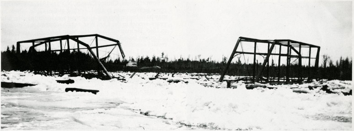
Ice and logs took out the bridge across the Flambeau River at the Vinette farm on April 14, 1906. Ice carried the bridge all the way to Ladysmith. It broke up on the booms of the Menasha Wooden Ware Co. before it reached the dam.
