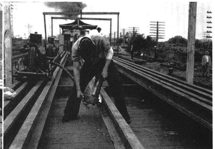
Left: Inside the welder car. The flash that gives part of its name to the electric flash butt welding process. Right: Fillet grinder. (On third flat car). Upset metal at "fillet," immediately below rail head, and upset metal immediately above base is removed. This is done to eliminate possibility of a fatigue fracture developing at these points of compression and tension when rail is carrying load in track.
