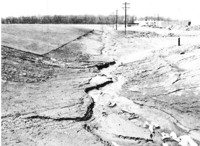
Figure 61 SOIL EROSION DURING HIGHWAY CONSTRUCTION
