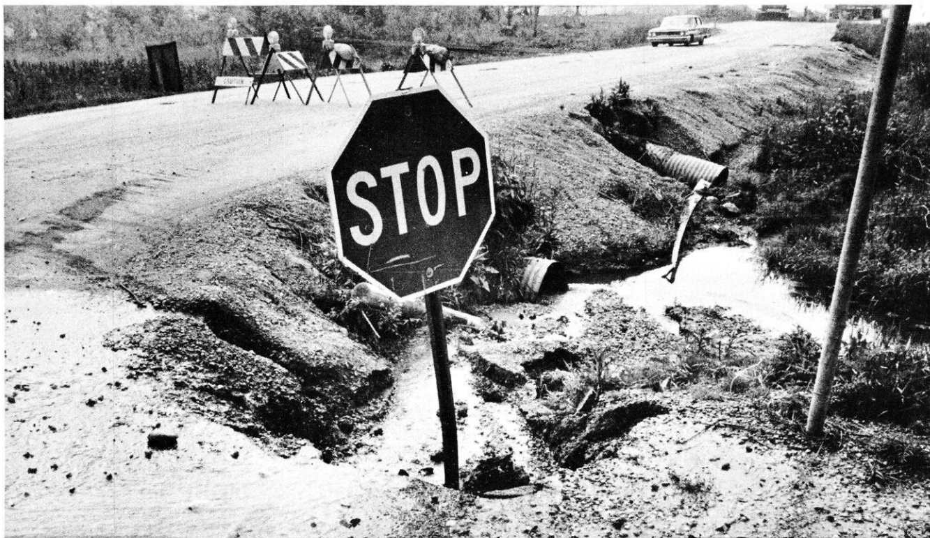
Figure 61 SOIL EROSION DURING HIGHWAY CONSTRUCTION
