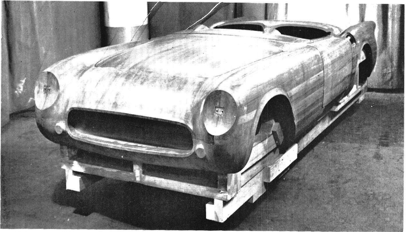
This wood model is composed of a separate model for each panel. It is constructed in such a manner as to also make it suitable for use in making the tools for production.
