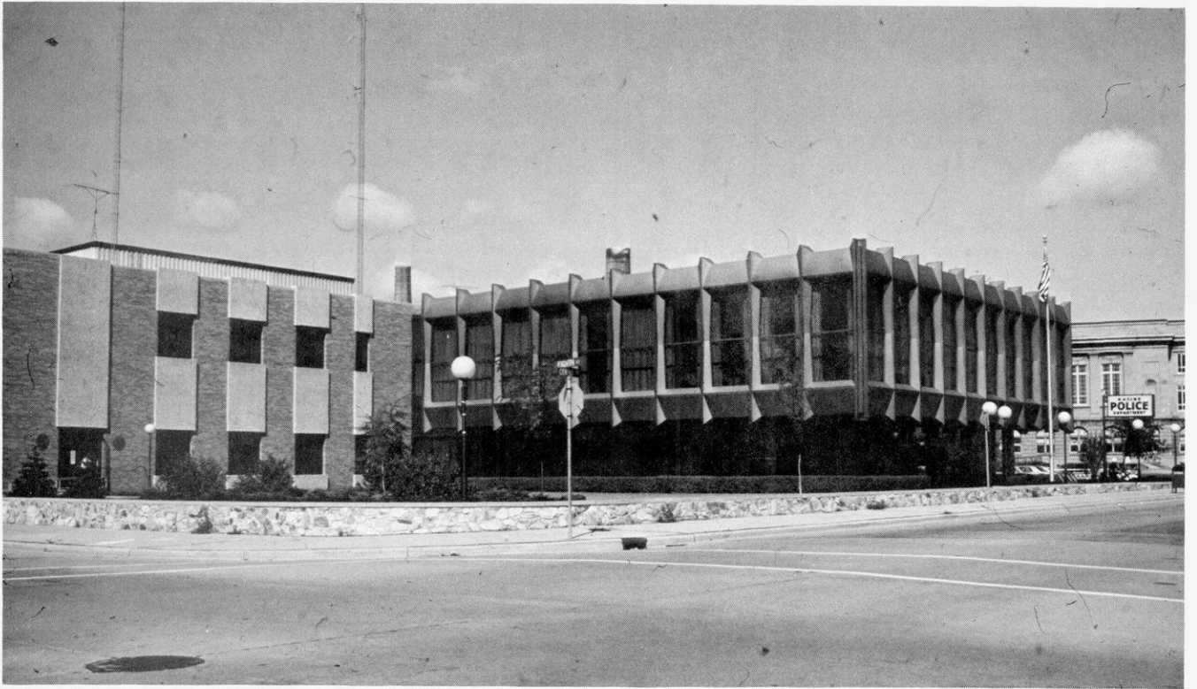
CITY OF RACINE PUBLIC SAFETY BUILDING
