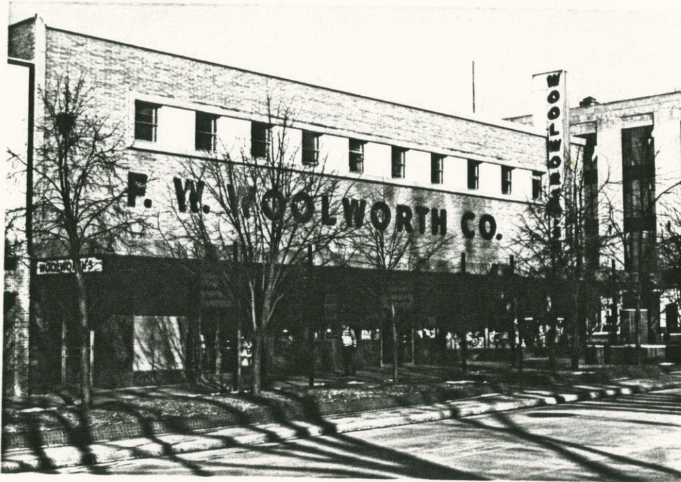
2 West Mifflin Street
