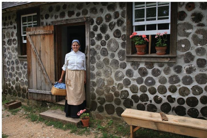
Below: The Kruza house at Old World Wisconsin is an example of a Polish farmstead from the late 19th century. It is an example of stove-wood construction, a European building technique wherein logs are cut into short, uniform sections and stacked to resemble piles of firewood. (Wisconsin Historical Society)
