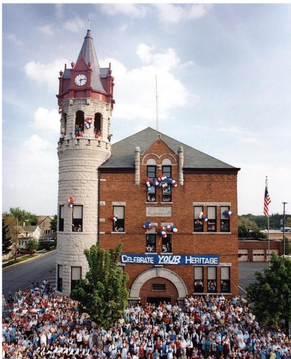
The key to the renovation of the Stoughton Opera House was a spirit of civic volunteerism, a phased restoration plan, and persistent fund-raising efforts. The refurbished theater was rededicated on February 22, 2001 – the 100th anniversary of its original opening. (Wisconsin Historical Society)
