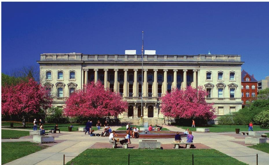
The Wisconsin Historical Society headquarters building, Madison, Wisconsin. (Wisconsin Historical Society photo by Robert Granflaten)
