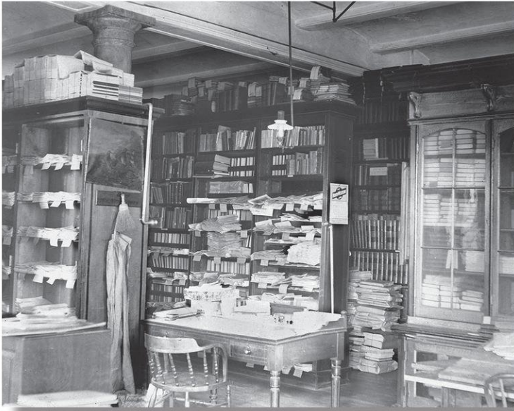
Stacks of the society library in 1898, when the society occupied rooms in the third Capitol building. At one time, gas light fixtures were used in this space, allowing an open flame to burn perilously close to flammable items like the newspaper collection. (WHi Image ID 23287)
