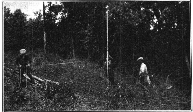
CROSS-SECTIONING ON RAILWAY WORK:
