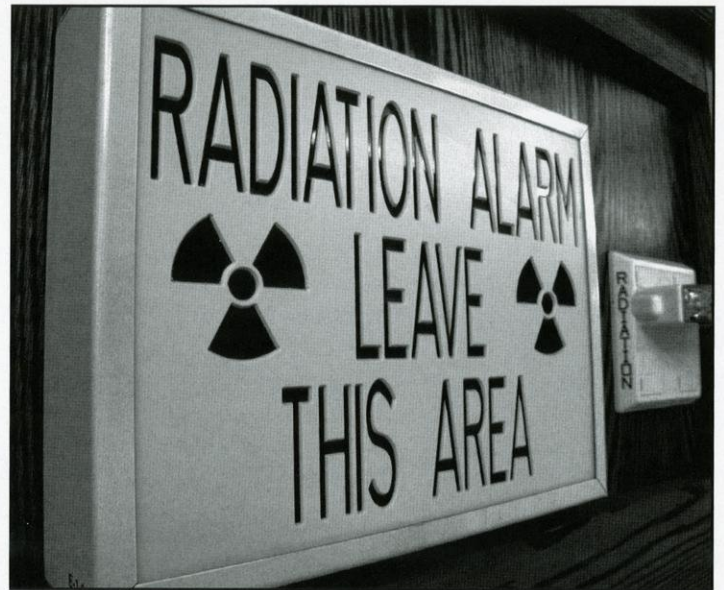
Signs in the Mechanical Engineering building light up to notify occupants if radiation is leaked from the research reactor.
