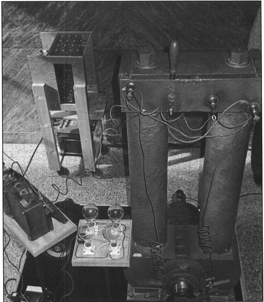
The Edison generator is enclosed in a glass case in the Electrical Engineering lobby.
