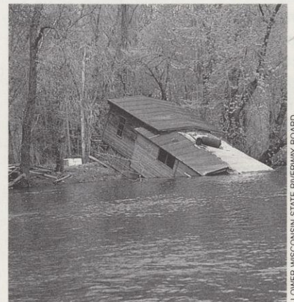
Eyesores like this dilapidated, abandoned house built in the river floodplain prompted a plan to protect the river's scenic beauty.
