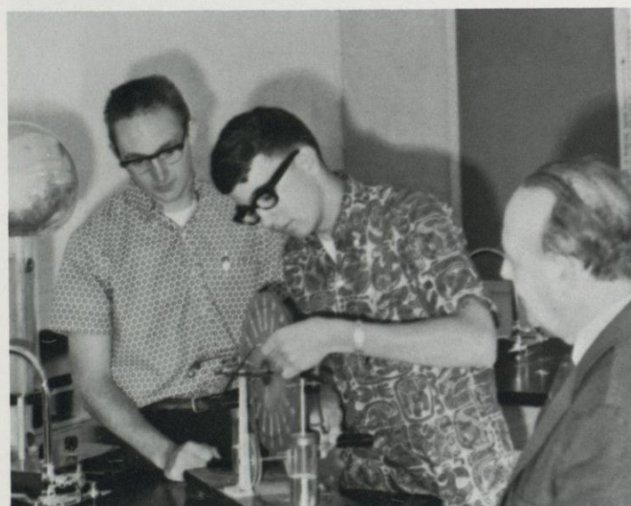
Randy and Dave are fixing the brushes on a generator in Physics class.
