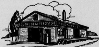
Storage capacity 250 tons sacked feed Saukville, Wisconsin Near C. M. & St. P. Depot
