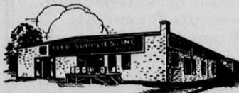
Storage capacity 1800 tons sacked feed NORTH MILWAUKEE STORE 3328 W. Cameron Ave. Opposite C. M. St. Paul Depot Telephone HI 11top 6930
