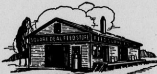
Storage capacity 250 tons sacked feed Saukville, Wisconsin Near C. M. & St. P. Depot
