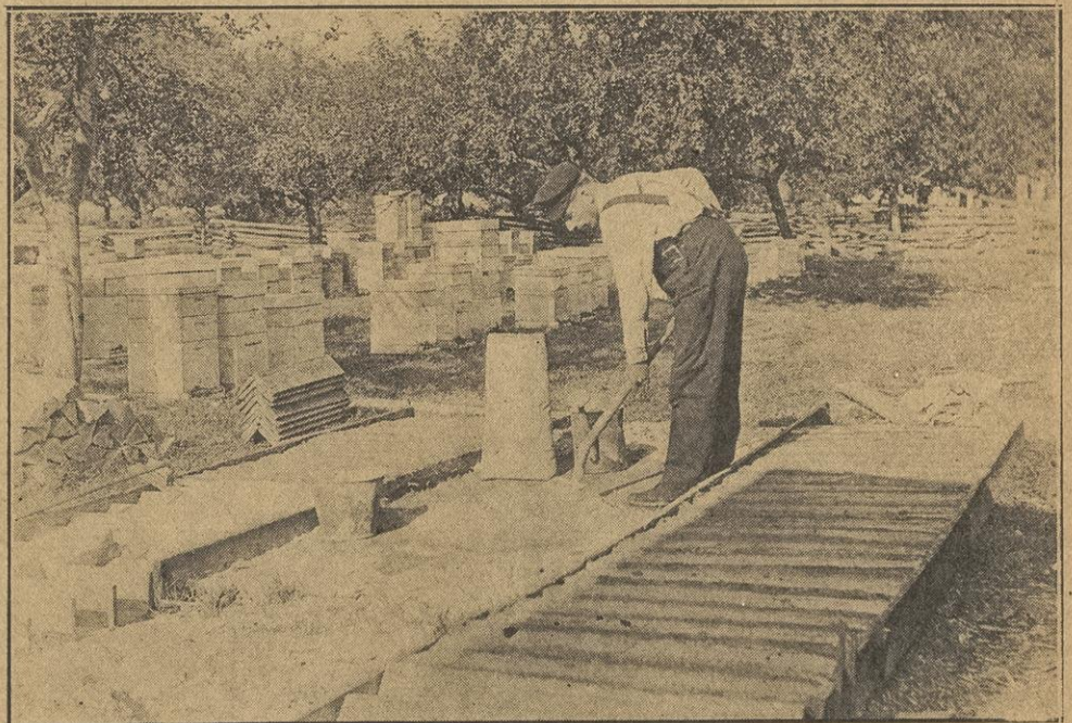
Making cement blocks for hive stands in the apiary of G. A. Deadman, Brussels, Ont.
