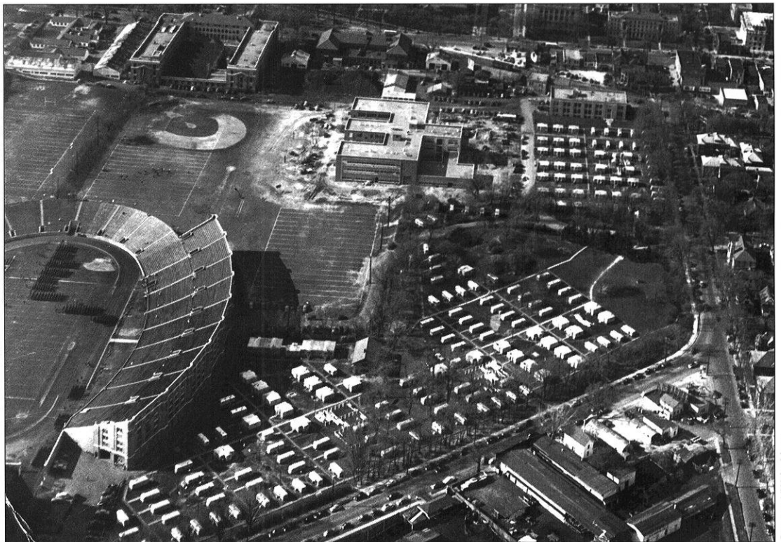
A photo of the engineering campus taken in the early 1950's. Notice the half-finished Engineering Hall (the backwards E-shaped building) and the plethora of temporary buildings.
