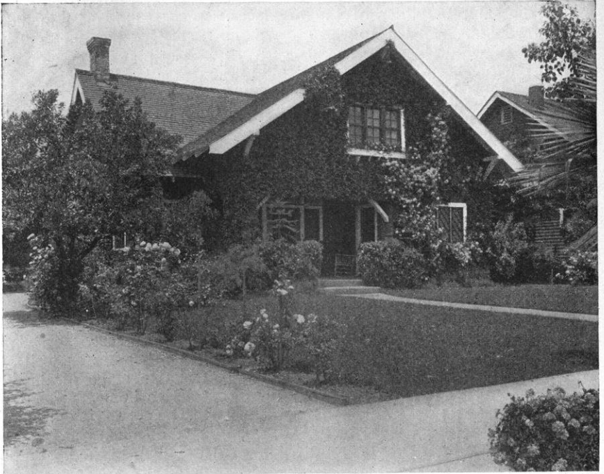
A CALIFORNIA COTTAGE OF INTERESTING DETAIL BUILT AT A COST OF ABOUT $2,800
