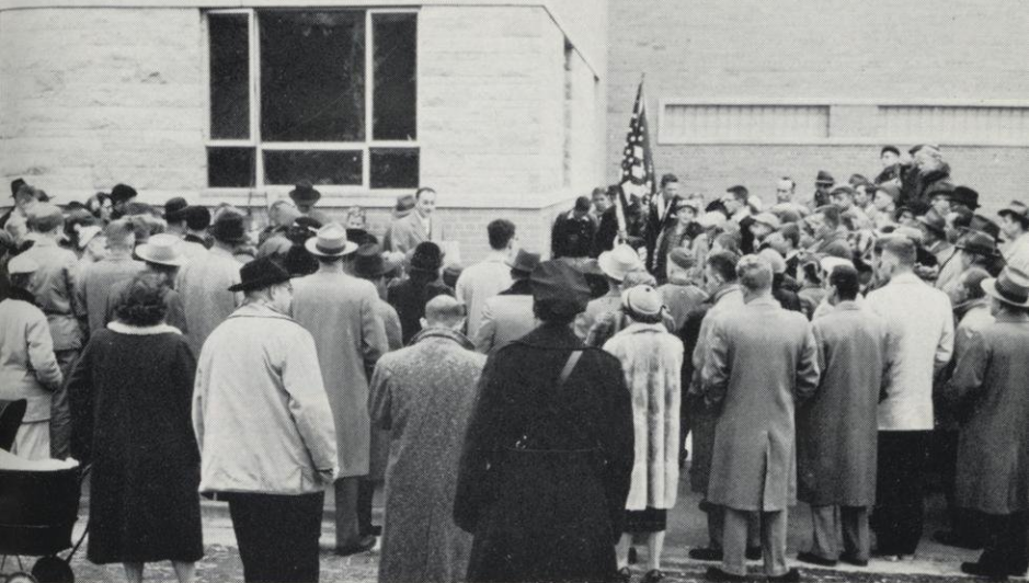
Laying of the cornerstone, November 18, 1956. Remarks by Gordon Altenhofen.
