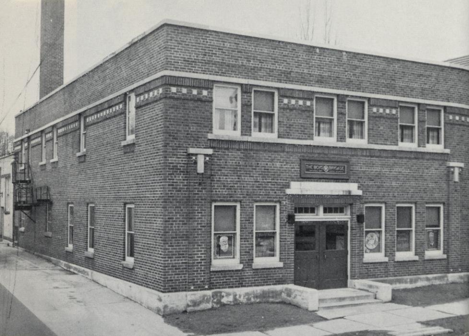
The Danke Building purchased in 1928. At the rear, the gymnasium built in 1938.
