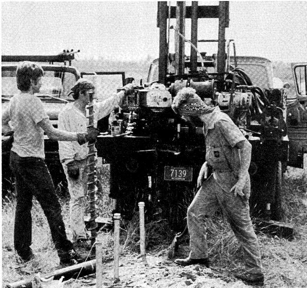
Staff members of the Geological and Natural History Survey installed monitoring wells near Wisconsin Rapids as part of a research project to measure long term variations in groundwater levels and the impact of agricultural chemical use on groundwater quality (photo courtesy of Wisconsin Geological and Natural History Survey).
