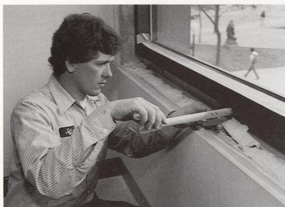
All windows in the building were replaced with insulated window units and argon gas-filled reflective glass, and fin-tubing was added to keep windows frost free.
