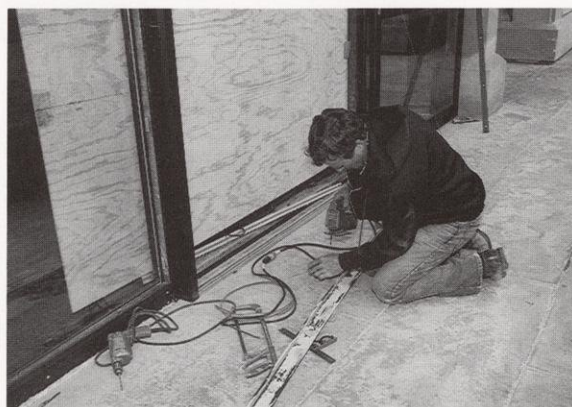
Vestibules were installed at the University Avenue and the Murray Street entrances to help stabilize interior temperature.
