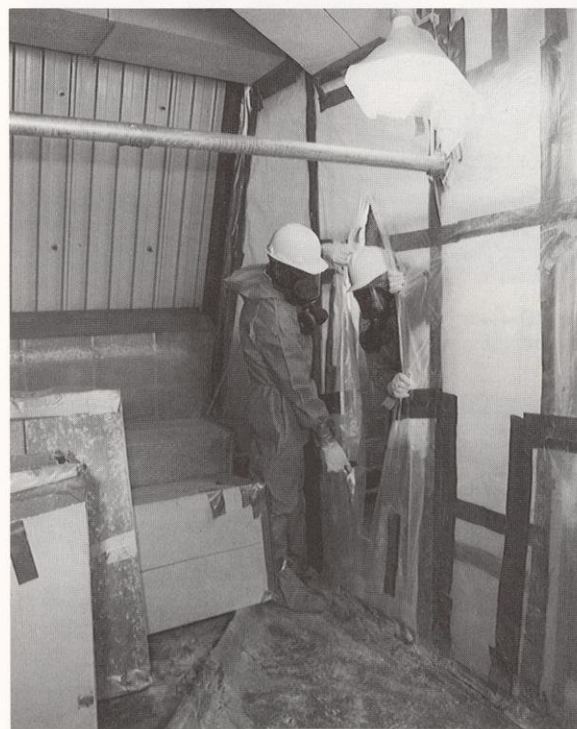
In the attic a seal was constructed to isolate the area of asbestos removal. Photo by Babboni's Creative Images, West Allis
