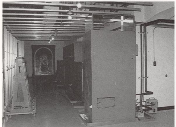
Temporary air conditioners were installed in the painting storage room to stabilize temperature while improvements were made to the heating, ventilating, and air conditioning systems in the attic.
