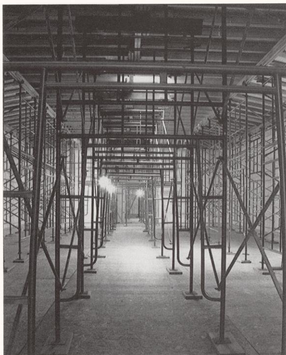
Scaffolds were installed in the fourth floor galleries to support ceilings on which people were working.
