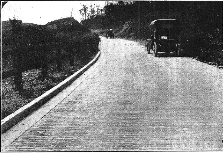
FIG. 3.—Warren Road, Ohio. Brick on Concrete Foundation.
