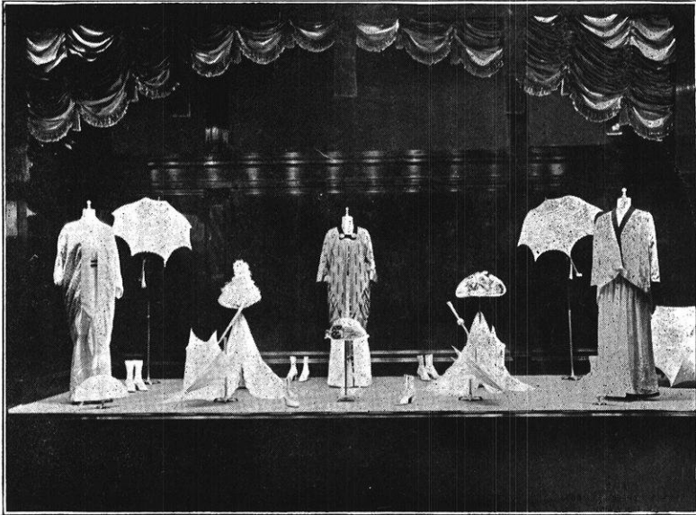
FIG. 6.— Correct window lighting from concealed sources. Equipment—100 watt tungsten lamps equipped with individual X-Ray No. 780 reflectors; units spaced on 18 inch centers.
