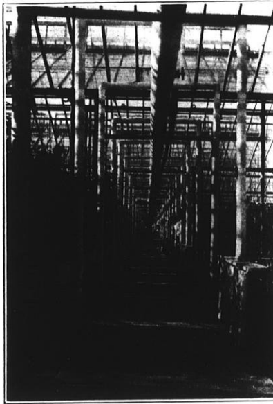
ACRES OF STEAM PIPES.
