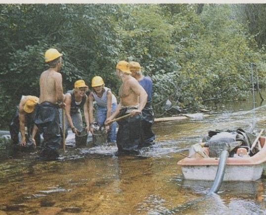
Foot by foot, YCC crews sandbag shallow streambanks to stem erosion, increase water flow and build better fishing habitat.
