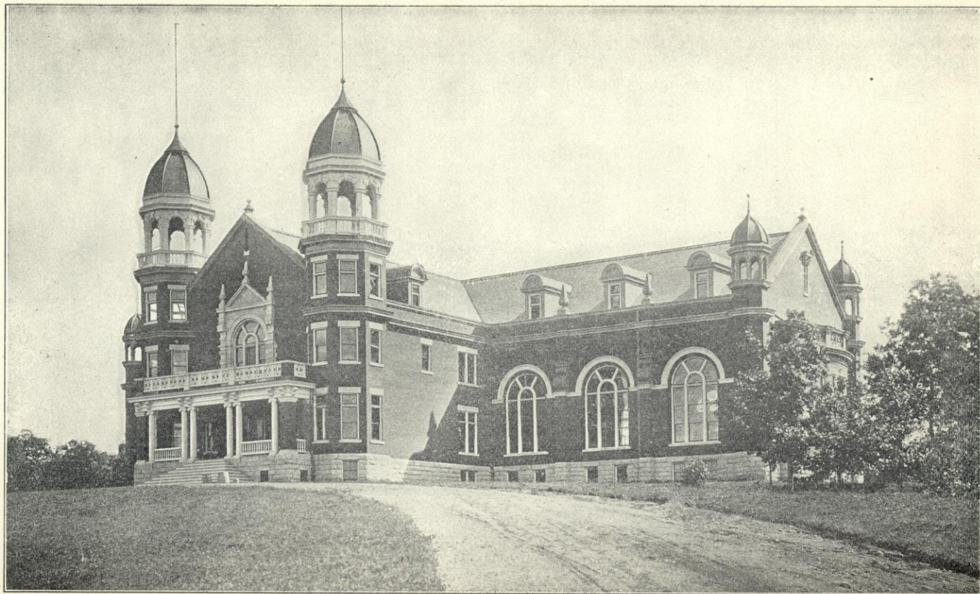
ADMINISTRATION BUILDING, HOME FOR FEEBLE MINDED, CHIPPEWA FALLS.
