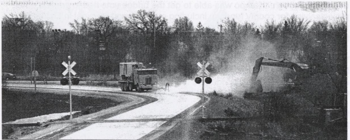
Workers putting final touches on the expanded STH 441, November 1991. Appleton Post-Crescent.
