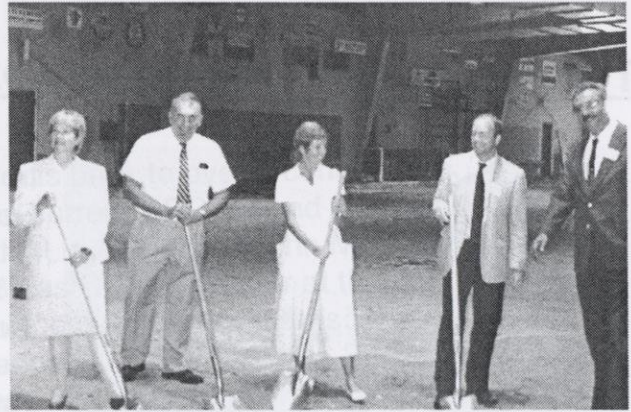
Groundbreaking for changing from a sand floor to a concrete floor. From left, Valerie Wylie, Paul Stevenson, Mary Grundman, David Berner and Corry Azzi. Tri-County Arena.
