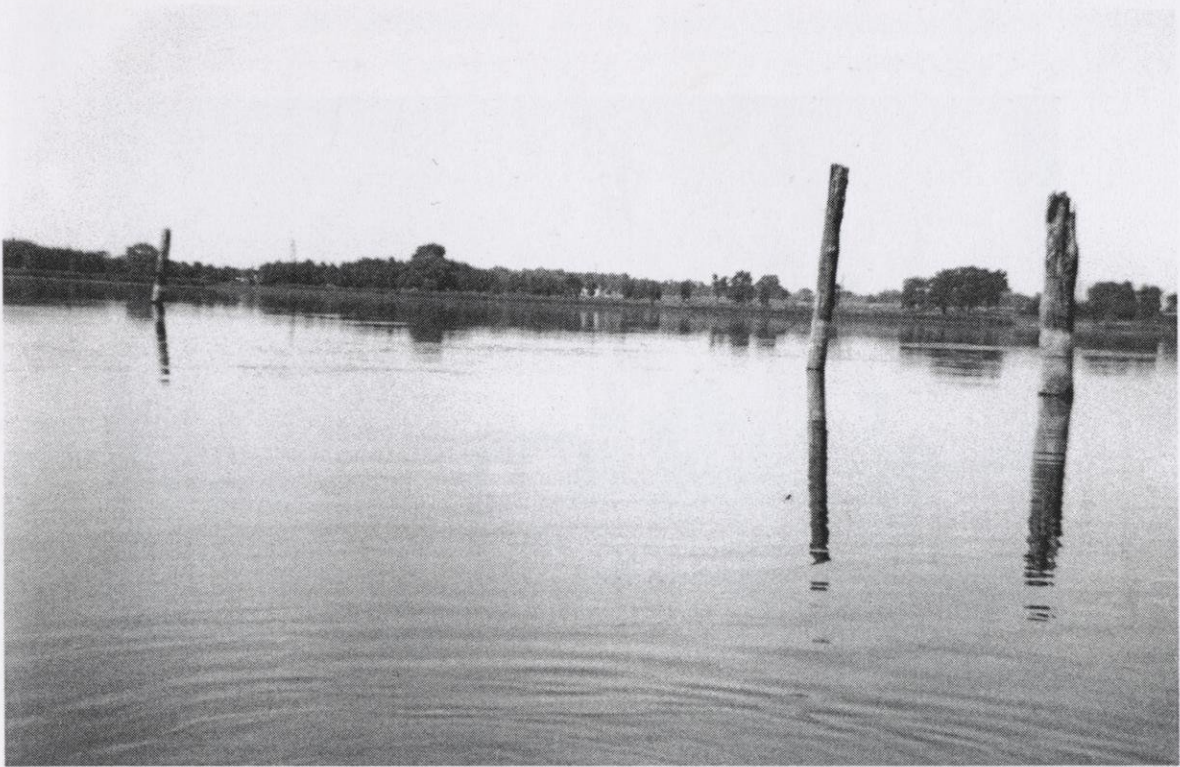
Photo from 1955 showing the old wood pilings that remained from the wagon bridge across Little Lake Butte des Morts. Richard Mason.
