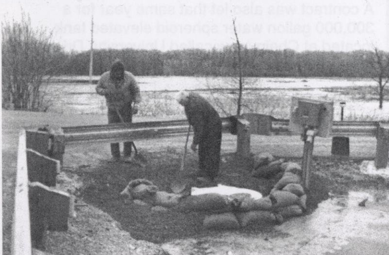
Stroebe Island lift station construction, 1978. Town of Menasha.
