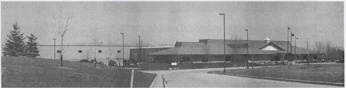
Town of Menasha Municipal Complex, housing administrative, police, park and recreation and street departments
