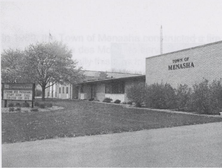
Former town hall on Valley Rd. now houses the east side fire station and a community center. Author.
