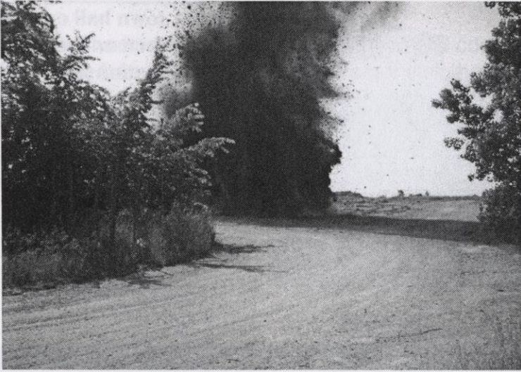
Demolition blasting for municipal complex, 1995. Town of Menasha.
