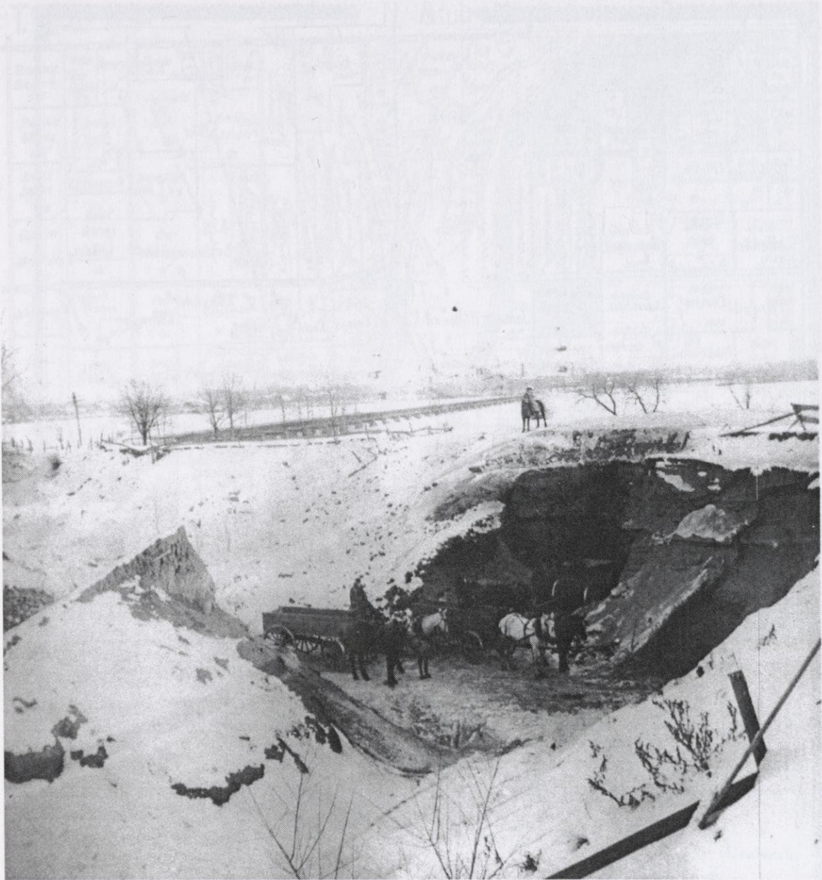
Quarry operations at the future site of Fritse Park, circa 1915. Neenah Public Library.
