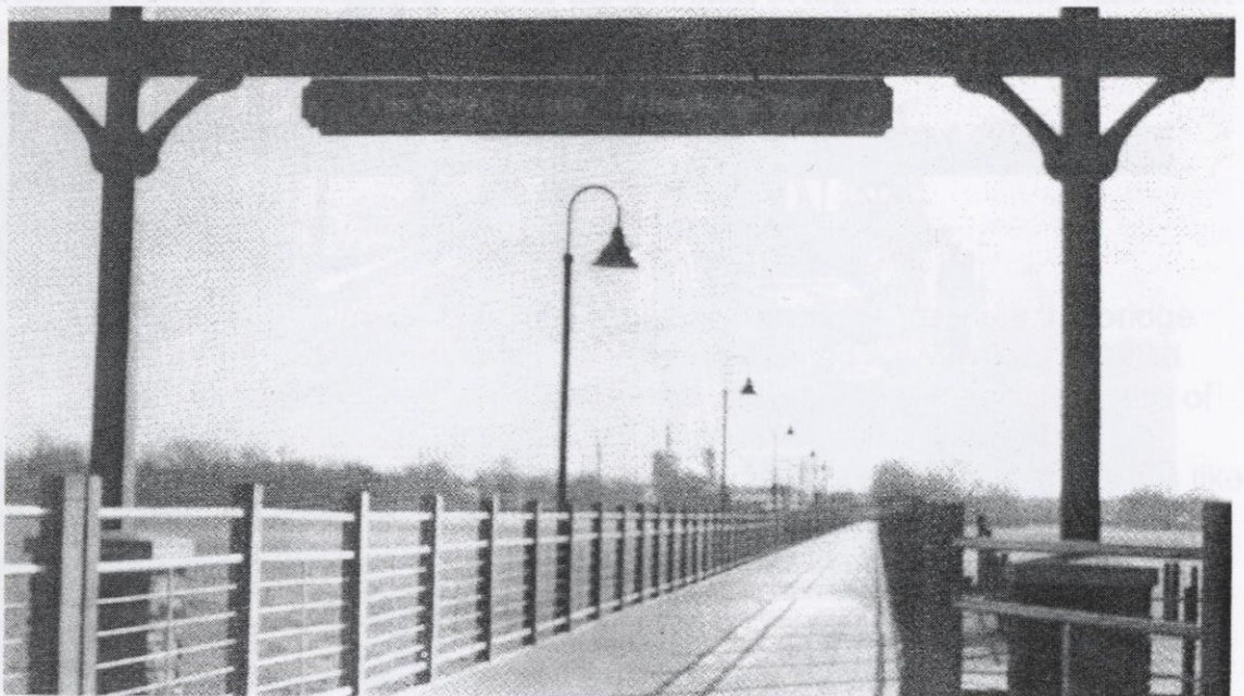
View from the Town of Menasha looking eastward towards the City of Menasha on the new Trestle Trail walking bridge. Larry Easton.
