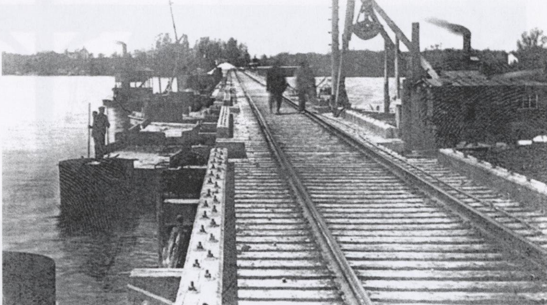
1910 photos showing the work progressing on the crossing. Neenah Public Library.
