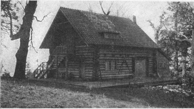
LOG CABIN WITH TILED ROOF.
