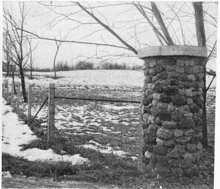
FENCE POSTS AND PILLAR CAPS OF CONCRETE.
