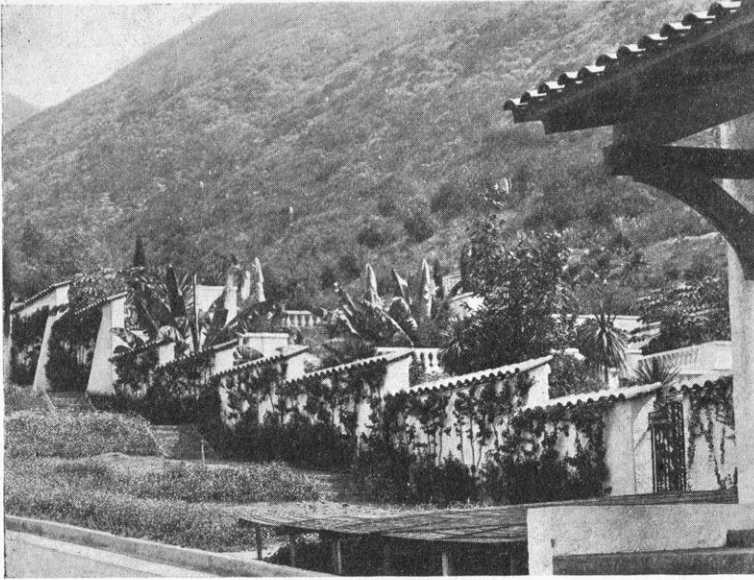
INTERESTING EFFECT OF A CONCRETE TERRACE.
