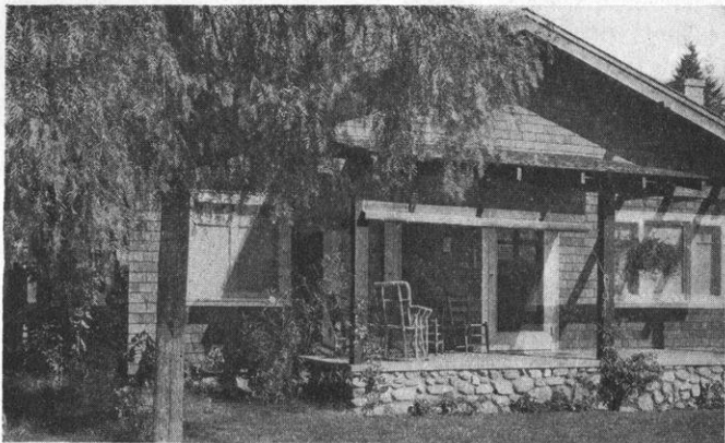
VERANDA WITH PART PERGOLA CONSTRUCTION.
