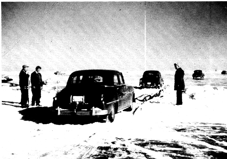
Bridges across pressure cracks allow vehicle travel over most of the lake.
