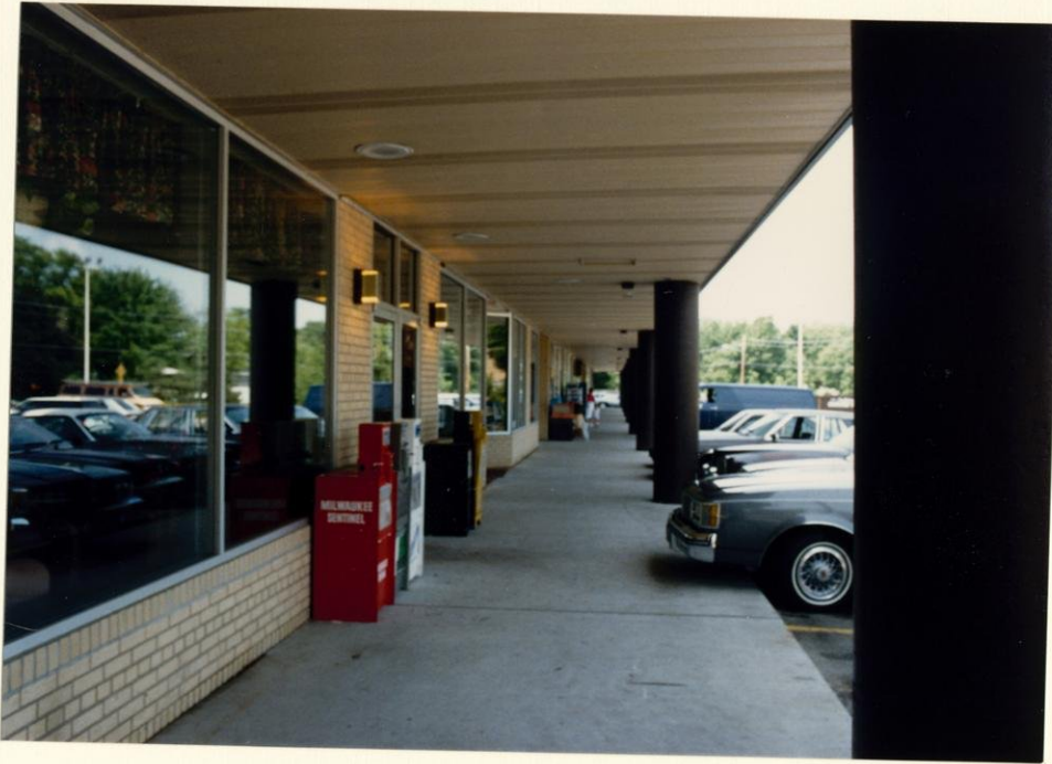
Modernizing Lake Edge Shopping Center has included a new look in the front facade such as substantial columns, and thermopane glass fronts.
