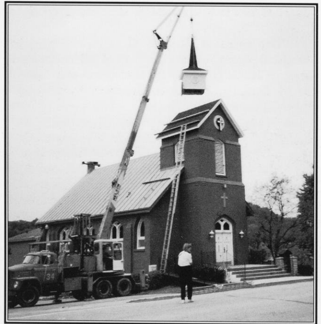
Above: The new steeple was placed atop the Zwingli U.C.C. on September 12, 1995. The steeple was built by John Beutler. -Courtesy of Walter Brink.
