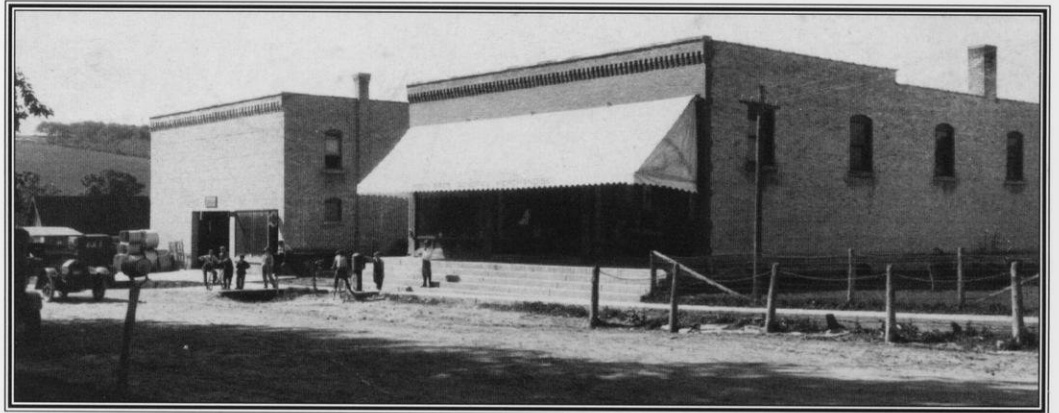
Below: Ad from the 1909 Mt. Vernon phone book. -Courtesy of the Mt. Horeb Area Historical Society, Inc.
